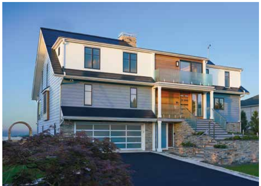
ABOVE: A combination of pitched and flat roofs and a blend of exterior materials give the home plenty of personality. The pitched roofs sport Tesla glass solar panels for energy efficiency. BELOW: Alder-trimmed doors fold out of the way, screen doors disappear into pockets, and the deck's railing is glass, all to maximize the indoor-outdoor connection.
